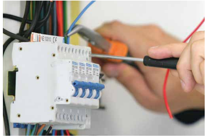
Covering Electrical & Data Cabling
