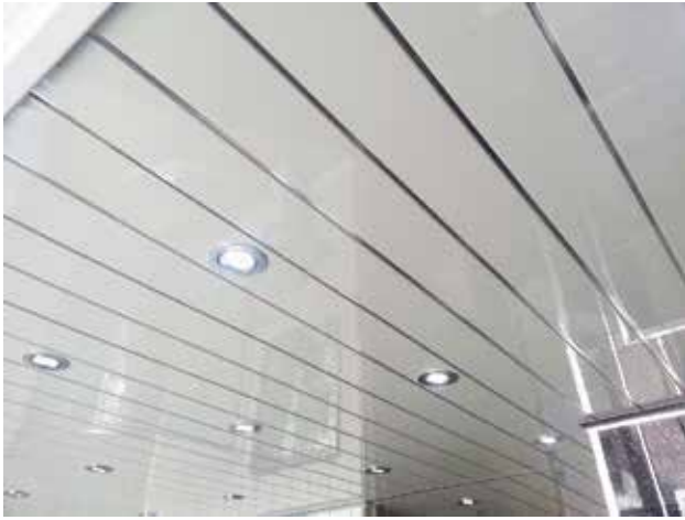
PVC False Ceiling
